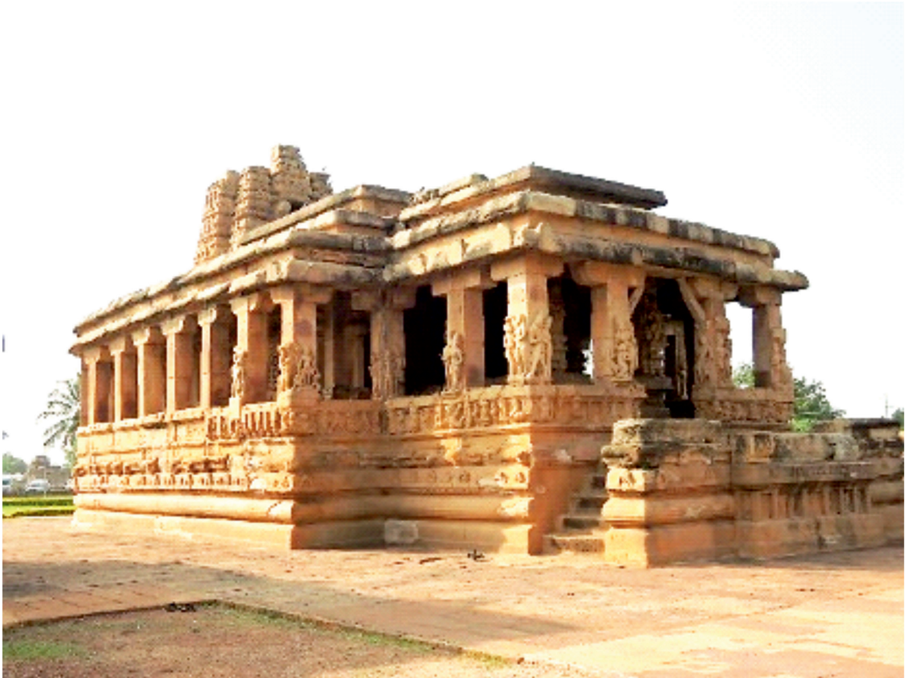
Figure 3: Durgi Gudi of Aihole in apsidal form made of sandstone
